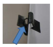
Flange of damper inserted here.
