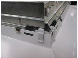
The flanges of the damper will fit <u>inside</u> the collar and be held in place by the clips.
